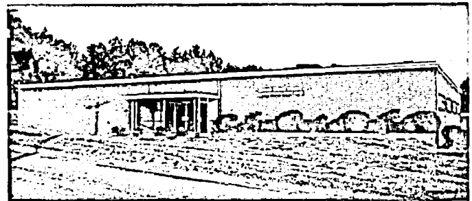
Energy and Environmental Research Annex
