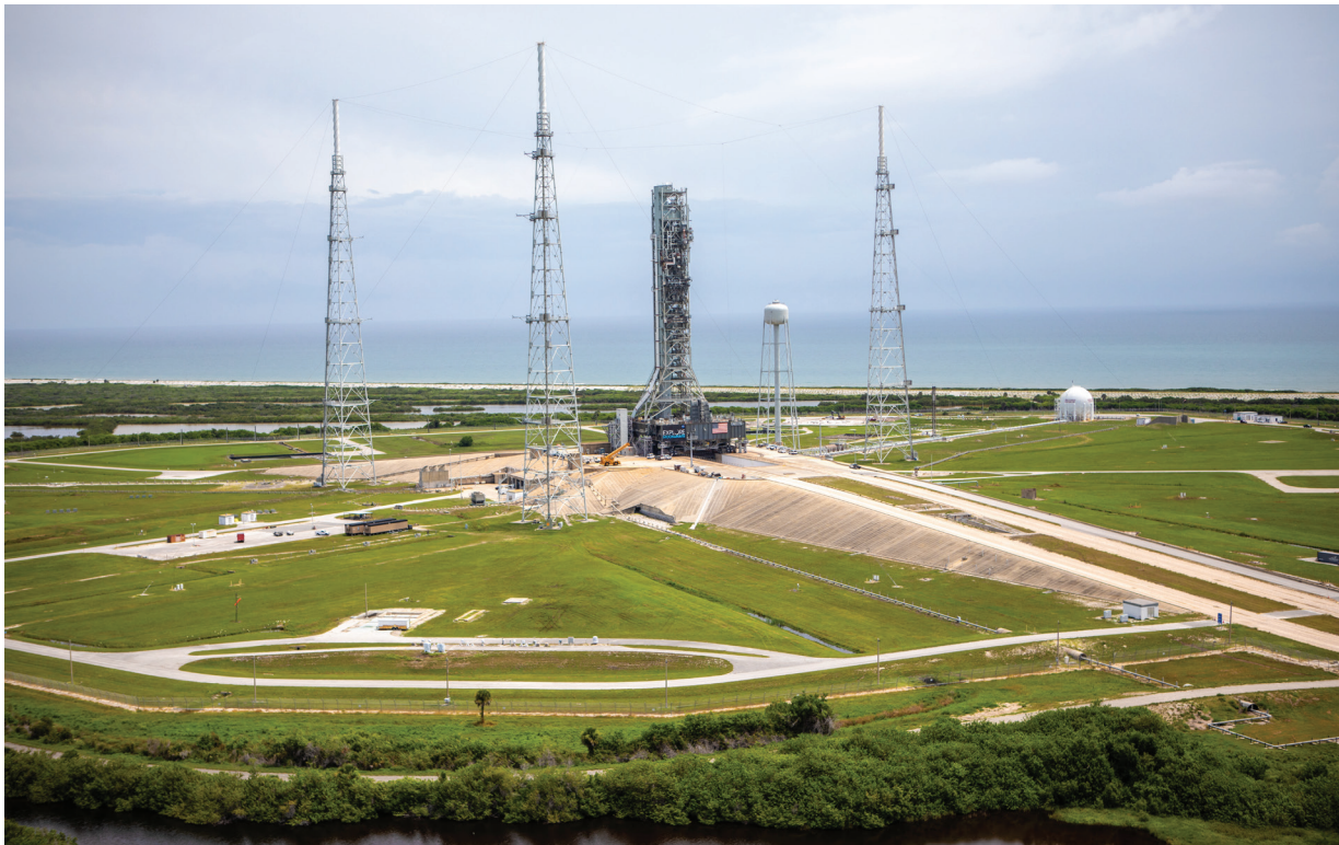
An aerial view of Launch Complex 39B at NASA's Kennedy Space Center in Florida. In view on the pad is the mobile launcher that will be used to launch the agency's Space Launch System with Orion spacecraft atop on Artemis missions. Photo credit: NASA/Kim Shiflett
