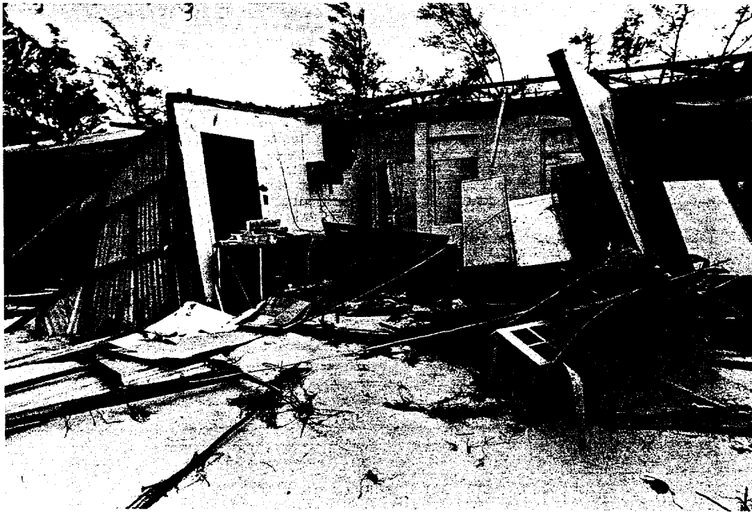
Figure 3-23-2. Many structures were extensively damaged by wind and water (Photo courtesy of Guam Publications, Inc.).
