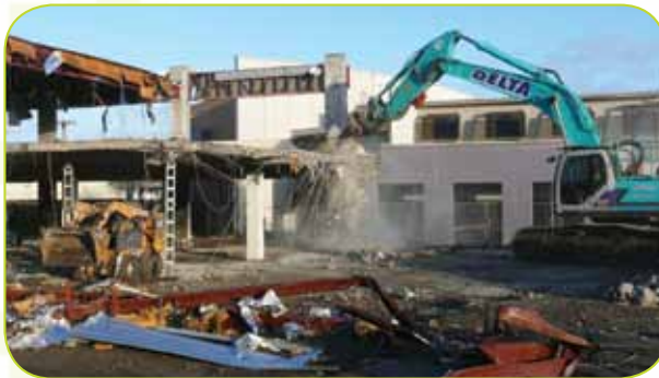
Demolishing the building at 81-85 Buckley Street Morwell, 2010
