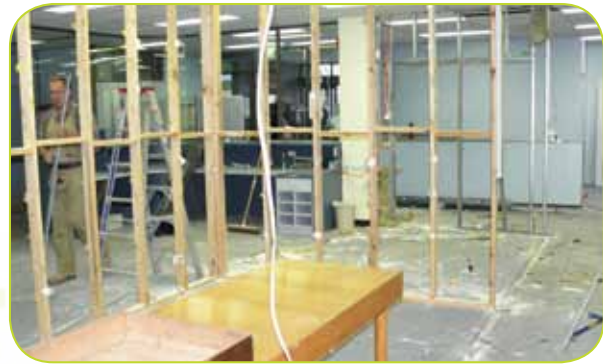
Upgrading the LCHS Buckley Street site Morwell, 2000
