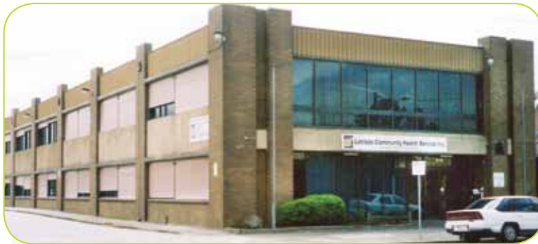
Former LCHS site at 81-85 Buckley Street Morwell
