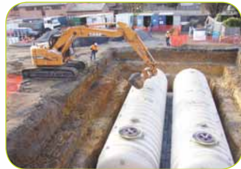
Installing underground water tanks at the Morwell redevelopment, 2009
