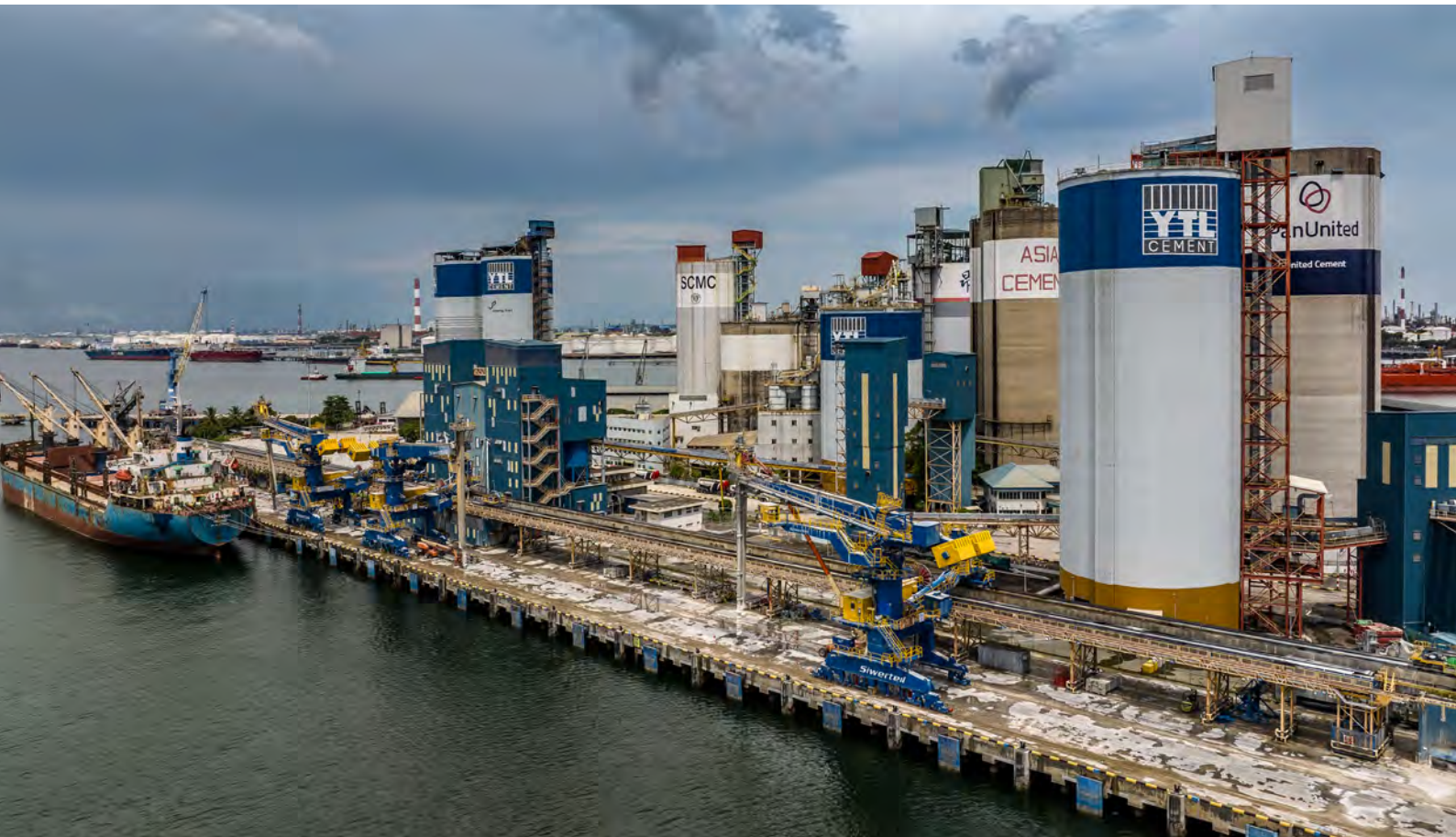
Below: Aerial view of Cement Terminal with new cement unloaders.
