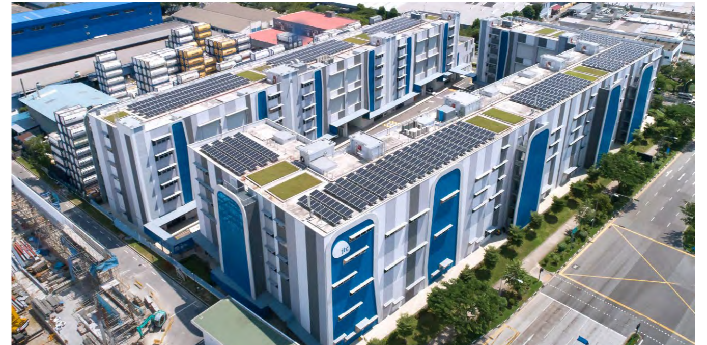
Aerial view of solar panels installed at the rooftop of JTC Space @ Gul
