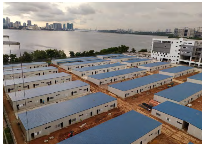
Aerial view of Quick Build Dormitories (QBD) that were set up in Kranji
