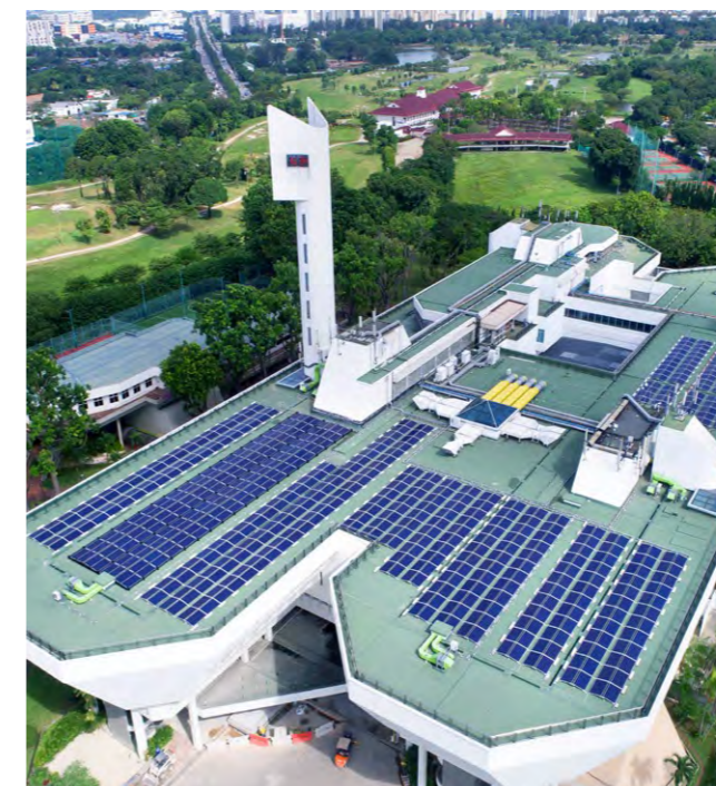
Aerial view of solar panels on the rooftops of JTC standard factories
