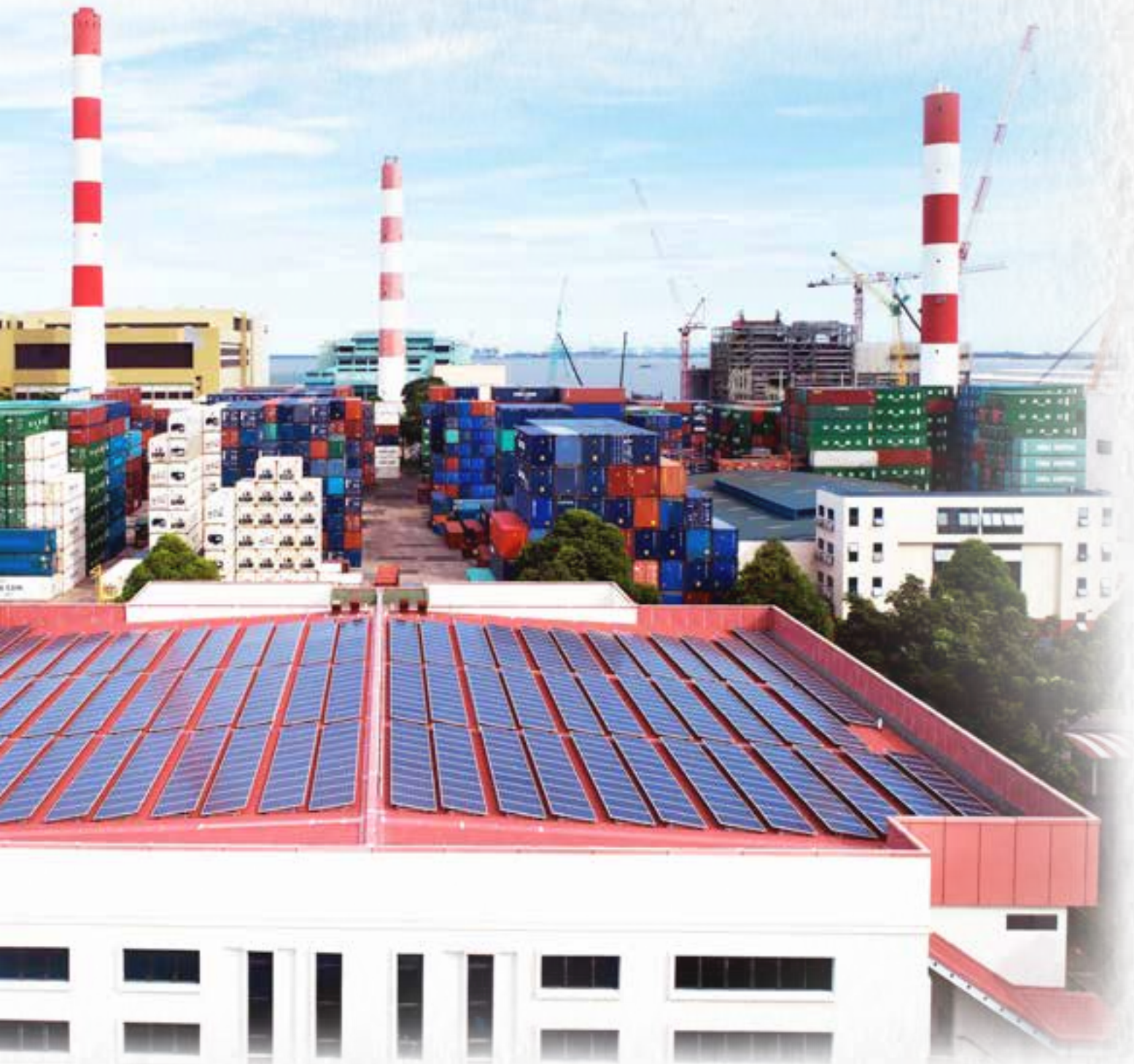
The SolarRoof test-bed included rooftops of JTC's standard factories in Tuas.
