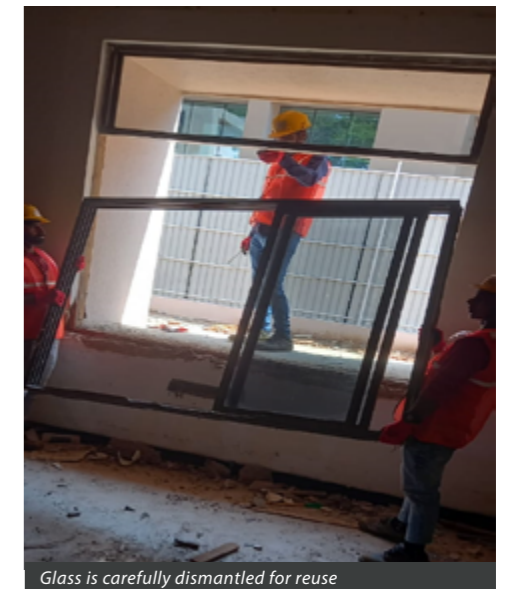
Glass is carefully dismantled for reuse
