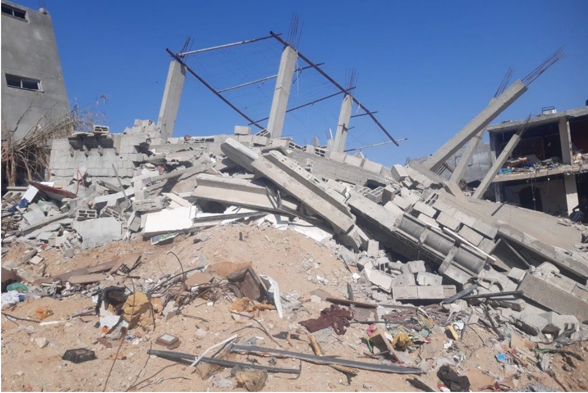
A photograph sent directly to Human Rights Watch researchers showing Sara's house reduced to rubble.
