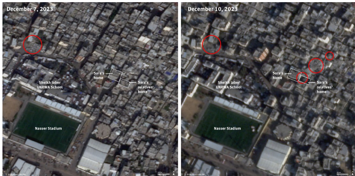
Before and after satellite imagery showing the location of the Israeli attack that destroyed Sara’s relatives’ home and severely damaged her own. The impact of two additional Israeli strikes carried out in the same timeframe are also visible on satellite imagery, dozens of meters northeast of Sara’s house. An earlier impact near the Sheikh Jaber UNRWA school was already visible in the December 7 image. © 2024 Planet Labs PBC. Right image: December 10, 2023. © 2024 Planet Labs PBC. Analysis and Graphics © 2024 Human Rights Watch
