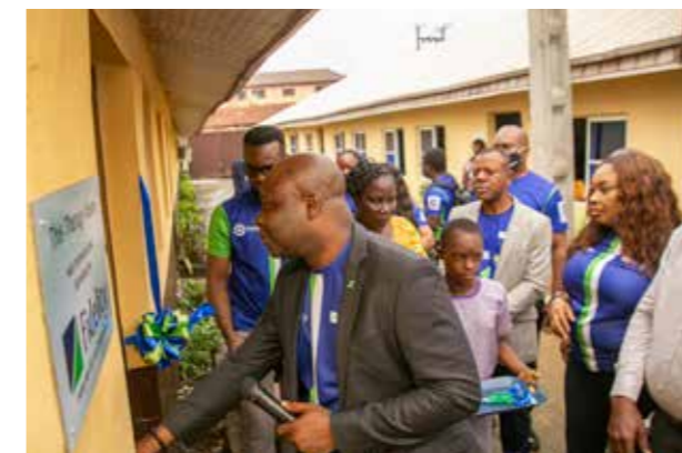
Internal Control Division renovates the Therapy room of the Modupe Cole Home.
