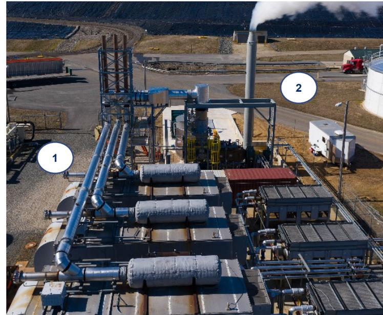
*(1) Hot generator exhaust gas is ducted together to provide thermal energy for evaporation in the Heartland Concentrator™ (2)*
