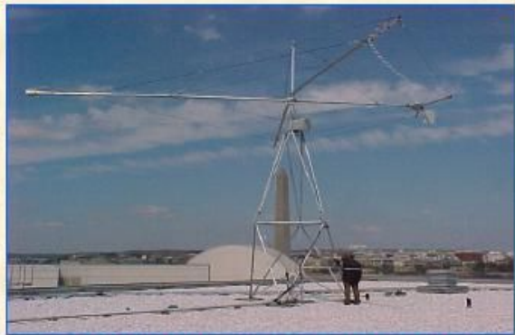
High Frequency Headquarters Building Roof Antenna Washington, DC
