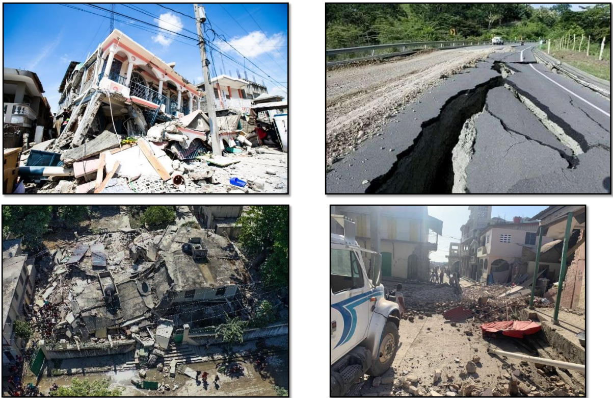
Figure 8 Damage caused due to M7.2 earthquake in Haiti. August 2021. Source: The New York Times, OCHA and Enfield Independent
