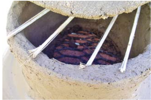
Pic 68. Before securing the base small twigs can be used for support.
