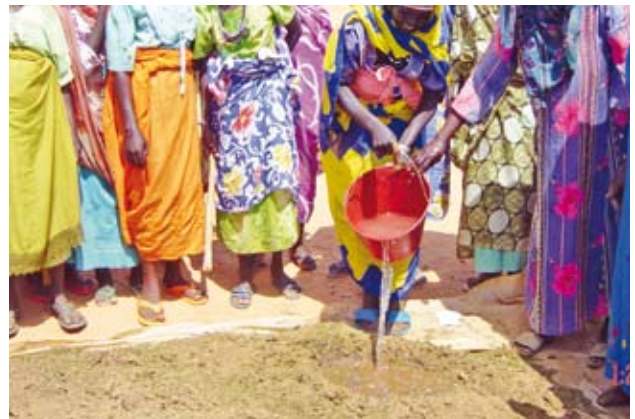
Pic 15. Enough water is added to form a sticky consistency.
