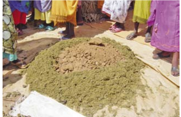
Pic 14. Soil is added to the dung approximately at a ratio of 3:2 (3 buckets of soil for every 2 buckets of dung)
