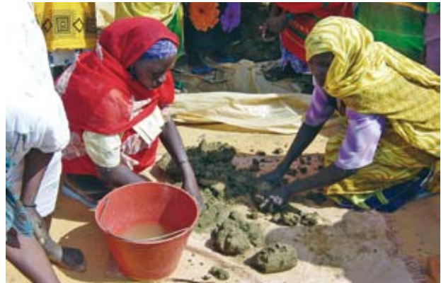
Pic 52. The clay is kneaded on a plastic bag.
