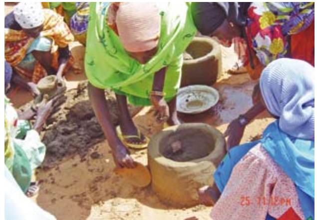
Pic 59. The pot is removed and using a scraper the surface of the stove is made smooth and left for about 1/2 hour in the sun before an exhaust hole is cut in the side with a sharp knife.
