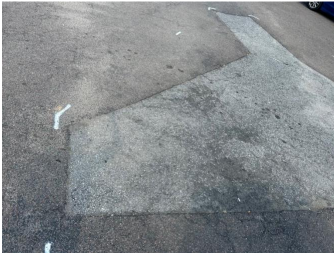
Aii Image 1: White-lining for road repair.
