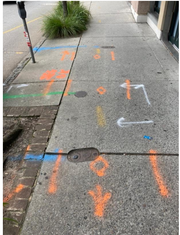
Aii Image 2: White-lining on a city sidewalk with other facility marks.
