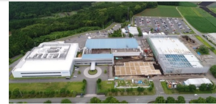
Expansion in Aso factory
