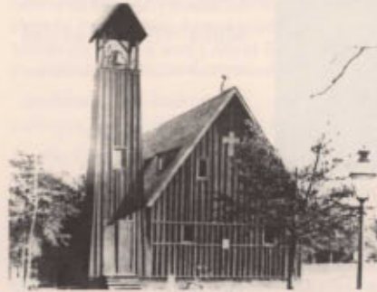
Trinity Protestant Episcopal Church, Piney Branch Road and Dahlia Street, NW (1893). An unusual board-and-batten redwood structure. Courtesy General Conference Seventh Day Adventist Church Archives.
