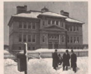
Takoma Elementary School, Piney Branch Road at Cedar Street, NW (1901, addition 1928, razed 1974). Courtesy Historic Takoma Inc Archives.
