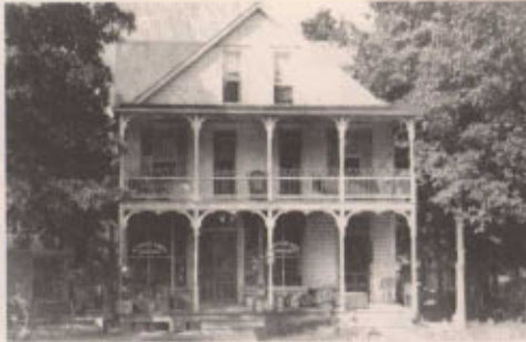
Favorite's Store, rebuilt on the site of the Issac Thomas store, burned in the fire of 1893. Courtesy Historic Takoma Inc Archives.
