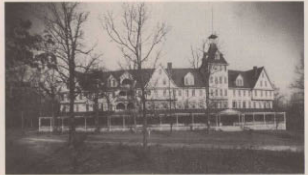
North Takoma Hotel, Takoma Avenue & Fenton Street (1892—burned 1908). 1906 photo courtesy Historic Takoma Inc Archives.
