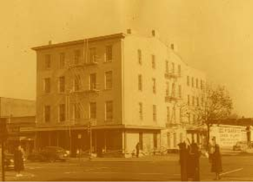
The former Thyson Mansion, which became the Salvation Army Corps No. 2, shown in 1950. HSW Photo.
