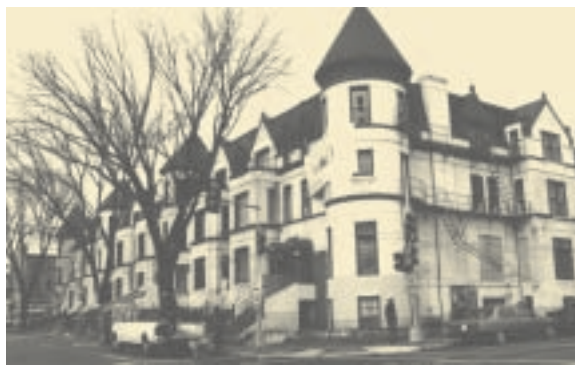
Left bottom: In 1890, the most prominent speculative development in the neighborhood was undertaken by noted Washington architect T.F. Schneider. To create distinction between each of the 53 rowhouses, Schneider alternated each building's form and size, applied detailing, and varied entrance styles. EHT Traceries, Inc.
