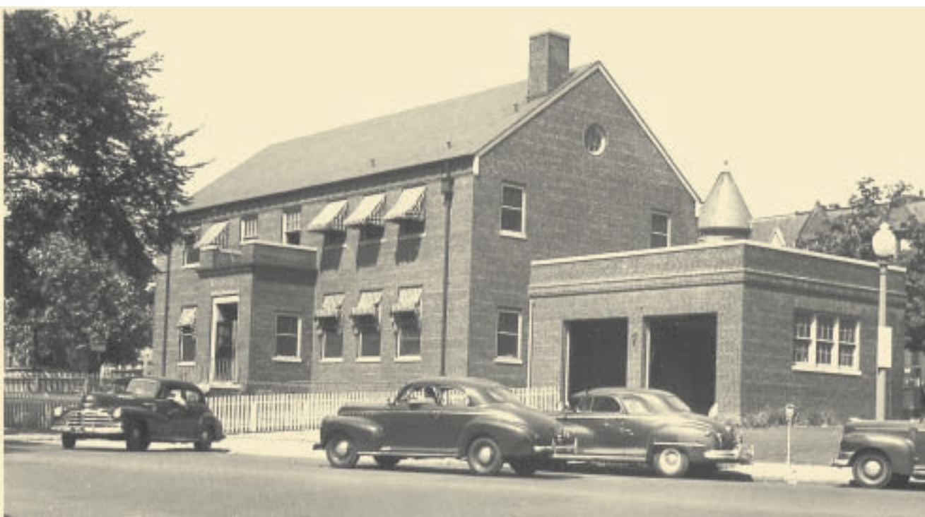
The Colonial Revival-styled District of Columbia Police Department, No. 2 Precinct Station at 5th & L Streets, N.W., was constructed in the mid-1930s. Sited on a triangular lot that historically was occupied by the Abbott School, the red brick Police Station is two stories in height with a corbelled brick cornice. Historical Society of Washington, D.C., 1949.
