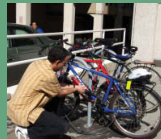
installing bike racks...
