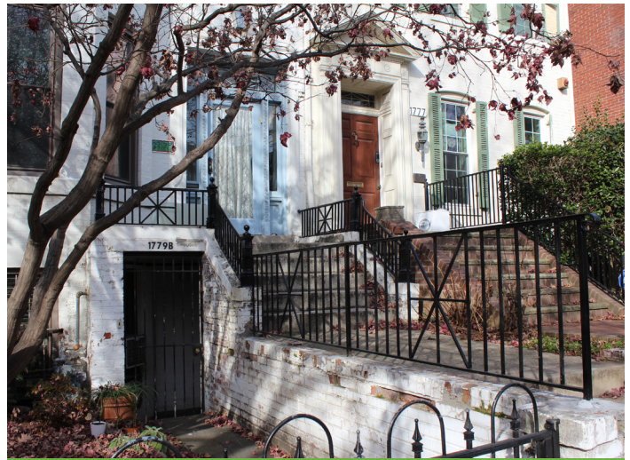
Attached Accessory Apartment in Basement of a Rowhouse
