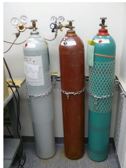
Gas cylinders chained to wall
