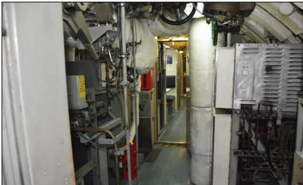
Turning around from the galley and looking aft, engineering is the next area.
