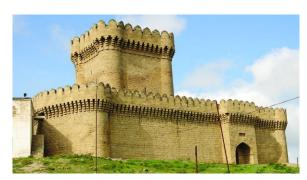
the 14th century. However, some researchers date the construction of the fortress to the 12th century. The inner courtyard of the fortress measures 28x10 meters. The outer walls of the fortress are reinforced with semicircular towers located at the corners and along the walls. A defensive platform is situated above the entrance to the Ramana castle. Unlike the three-tier structure typical of round donjons, the square-shaped donjon of the Ramana castle is divided into four tiers.
