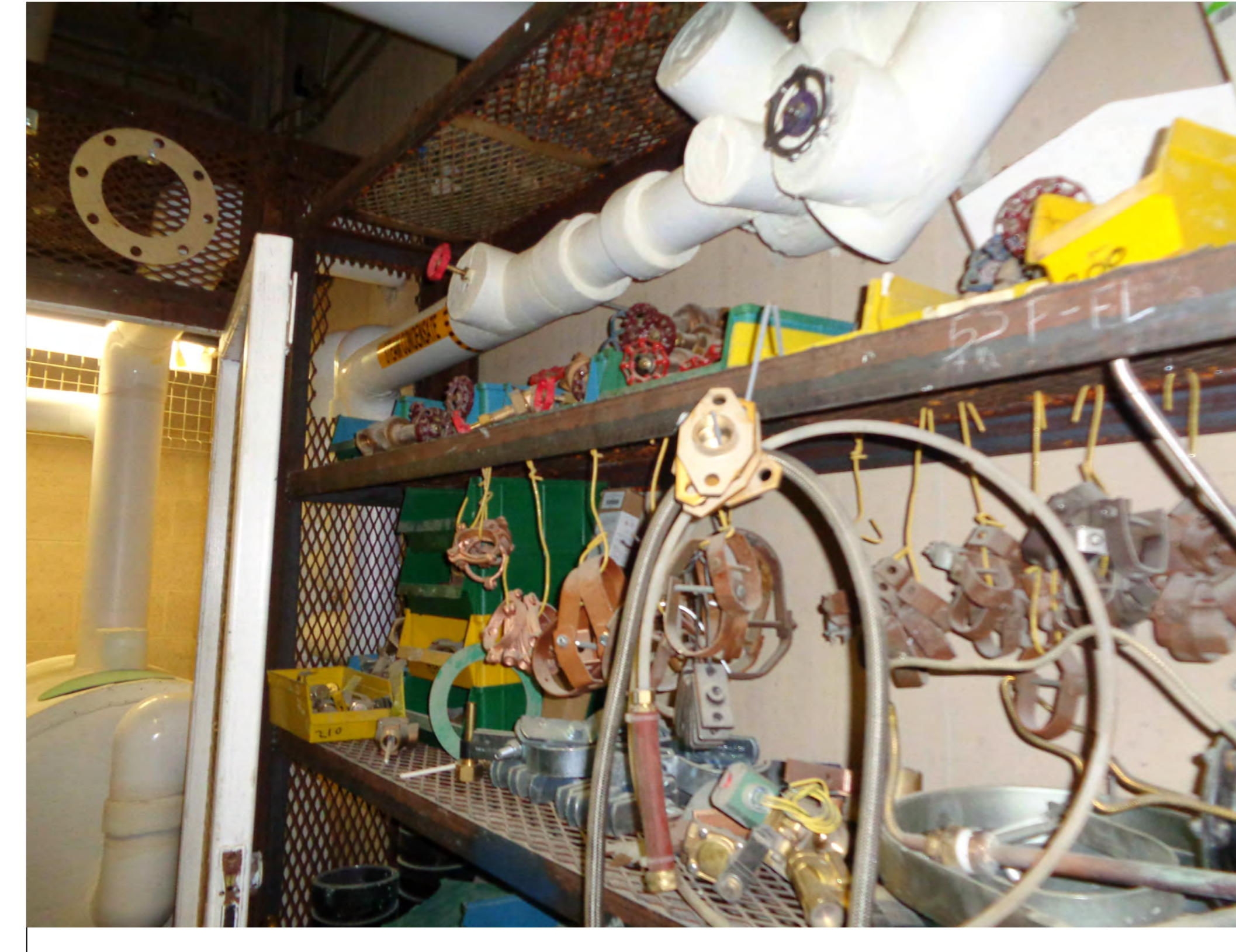
3 CONDENSATE PIPING AT FLASH TANK
