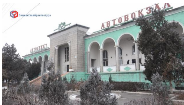
Figure 11. The Former Eastern Bus Terminal, built in 1962 on Zhibek Zholu Avenue. Photo: Bishkek Chief Architect's Office
