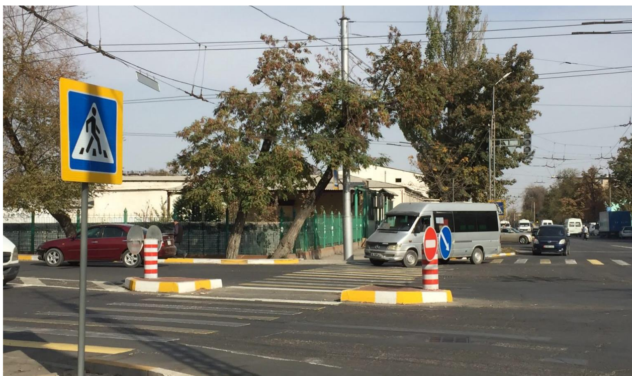
Figure 17. Installation of a pedestrian safety island. Photo: Road Safety NGO
