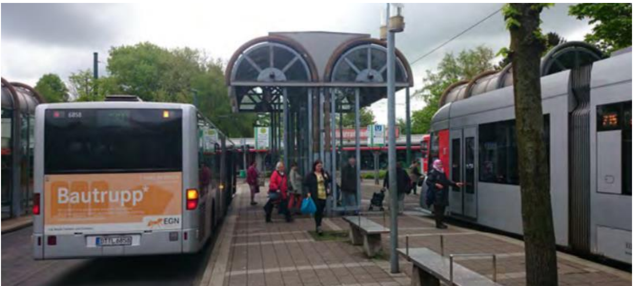
Figure 22. Cross-platform transfer from bus to tram in Dusseldorf, Germany. Source: Handbook on Sustainable Urban Mobility and Spatial Planning, UNECE, 2020
