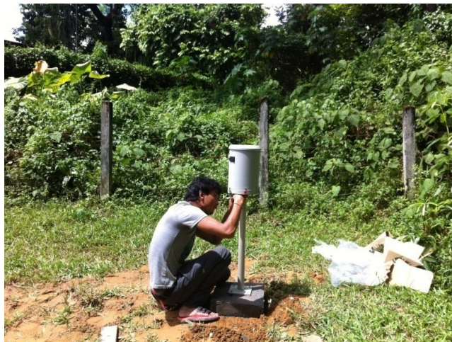
Figure 6.1: Installation of Automatic Rain gauge in Sylhet
